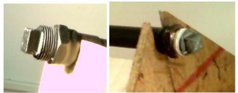
Figure 6: White pipe tape was used to help seal the plug. The first pictures shows the threads without pipe tape and the second picture shows the threads with the pipe tape. The pipe tape is intended to fill in the spaces between the threads.
